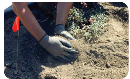
Create an irrigation berm to direct water to the root ball during establishment.
