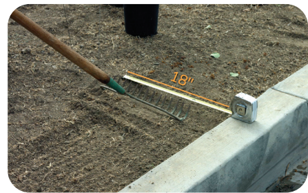
Level the surface in the 18" step-out area.
